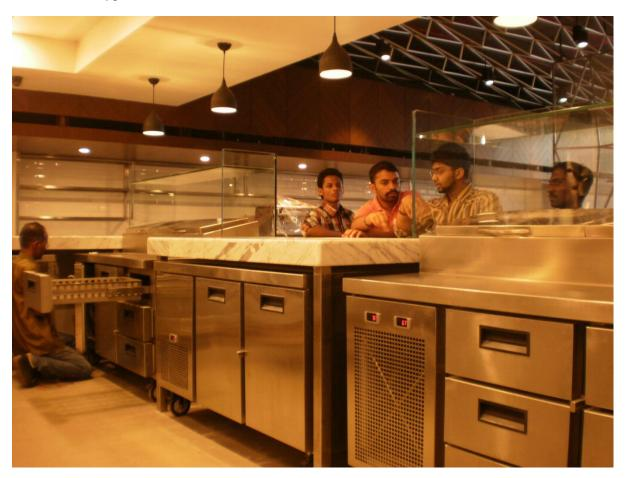
The prep stations come in two and three door versions, with chilled pans for ingredients mounted into their counter-tops and refrigerated cabinets below.
